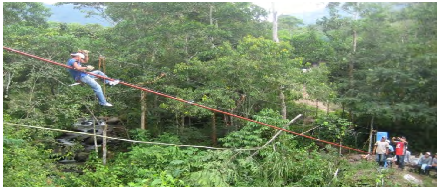
An ETAP student learning to put up a suspension pipe bridge with a sky hook.
